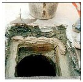
After twenty minutes the manhole cover can be put on, finishing with the final asphalt coat.
