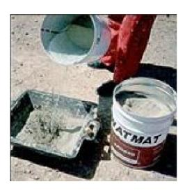
**Application:** Mix the required amount of WATMAT, place it around the perimeter of the hole, place the leveling tool on top and inside.
