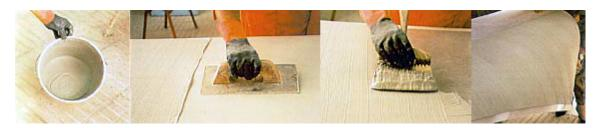
The surface to be coated must be sound, clean, free of all traces of paint, dust, grease, efflorescence, loose particles, form-stripping oils, gypsum plaster and curing compounds.
